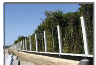
Noise barrier fixing
