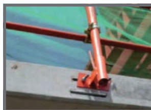
Guard rail fixing during the construction period
