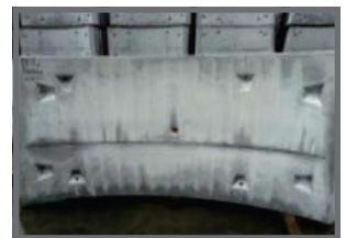
Finished precast segments with cast-in channels
