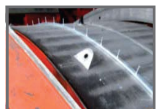
Channel installation into tunnel segment formwork
