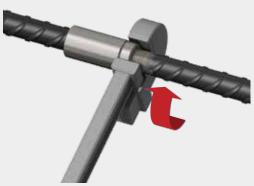
5 Hold the rebar in its required orientation and with a wrench tighten the locknut against the coupler. After tightening, the length of the exposed thread should be no more than half of the coupler length plus 4mm for sizes 20mm and below, or 6mm for sizes 25mm and above.
