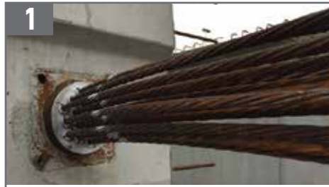
1 MK4 Post Tensioning System
