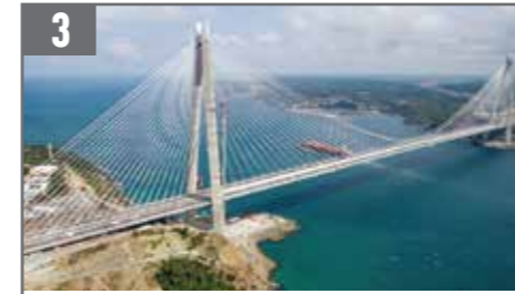
3 MK4 DMK Stay Cable System
