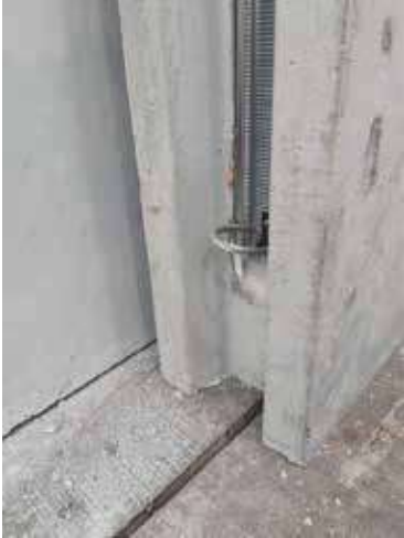
Images of precast walls with the wire ropes of MOMENT Multi Loop Box unfolded after casting.
