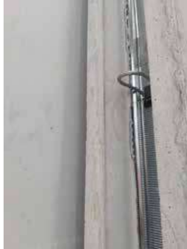
Images of precast walls with the wire ropes of MOMENT Multi Loop Box unfolded after casting.
