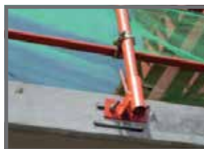
Guard rail fixing during the construction period
