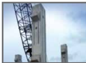
Vertically installed channels for pipe rack support
