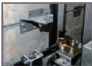
Elevator shaft - guide rail fixings
