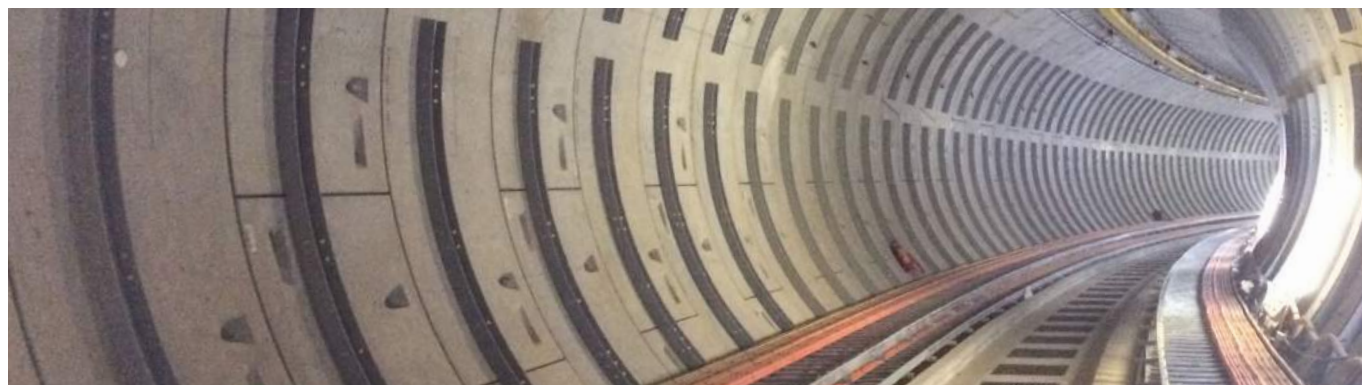
Singapore Power Transmission Cable Tunnel Project – HB-BZ
