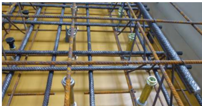
INSTALLATION OF FIXING ANCHORS
