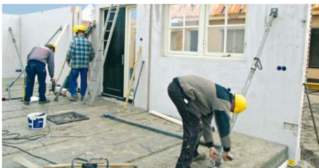
FIXING OF PROPS ON PRECAST ELEMENTS
