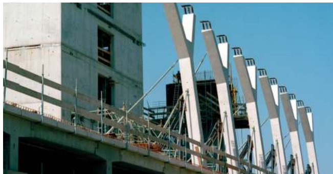
FIXING AND ADJUSTING PRECAST ELEMENTS
