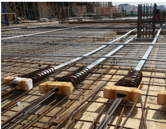
MPT Flat Slab System and flat duct being layed in position.
