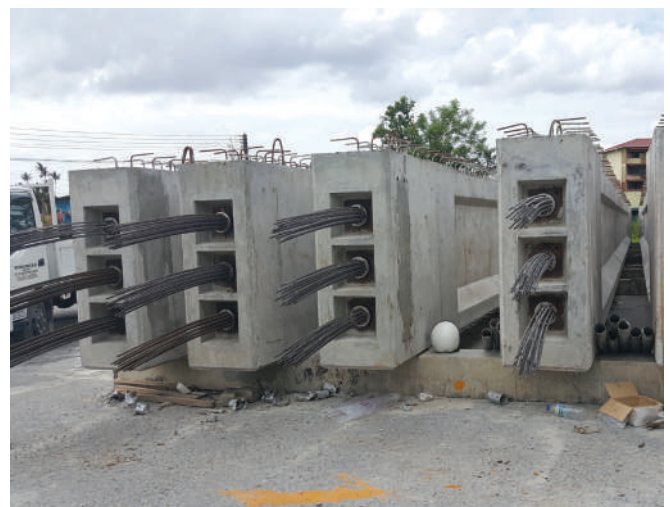
Post tensioning beams with anchor block and strand in place ready for stressing.
