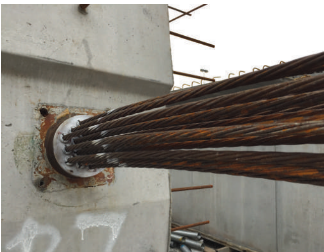
MPT Multistrand Round System on post tensioning beam.
