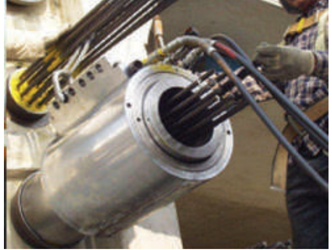
Multi Strand Stressing in progress. This process shall be done with caution.
