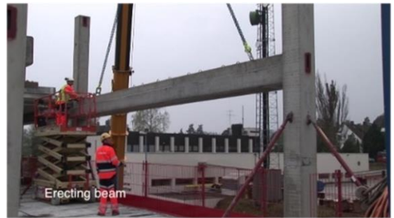
Precast Beam with BSF during erection
