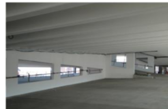
Precast T-Slab Installed with DTS for Multi-Storey Carpark
