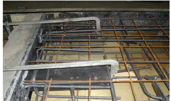
P2: TSS fasten with a clamp
