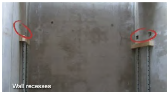
M4: Place the support for the landing, and adjust it to the right height.
