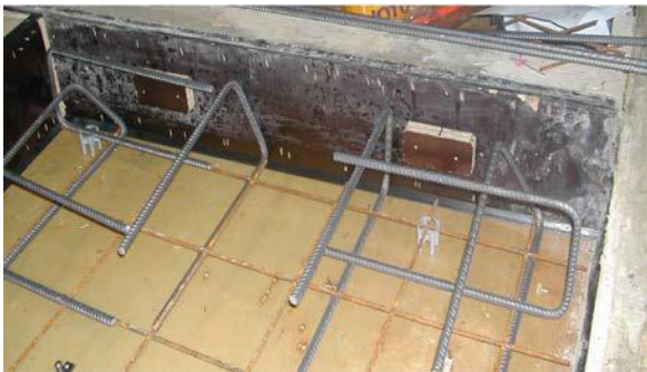
P1: Formwork with guiding piece
