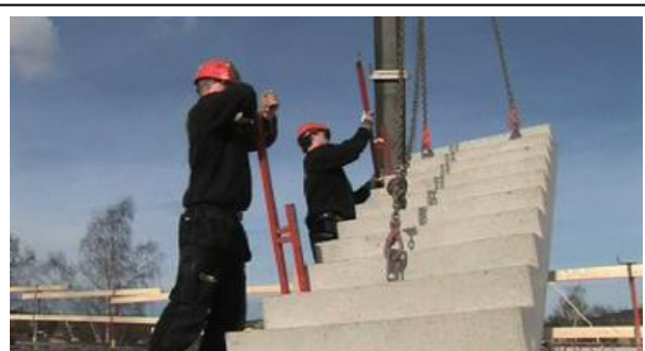
M18: Placing temporary railing to the stair.
