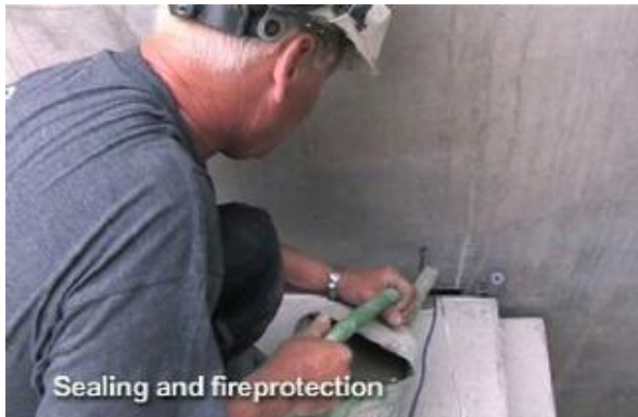
M13: Fill the gap with mortar
