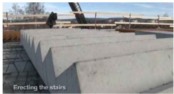
M16: Stair ready to be erect.
