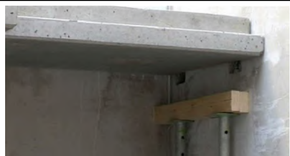
M6: Landing almost in the right position.
